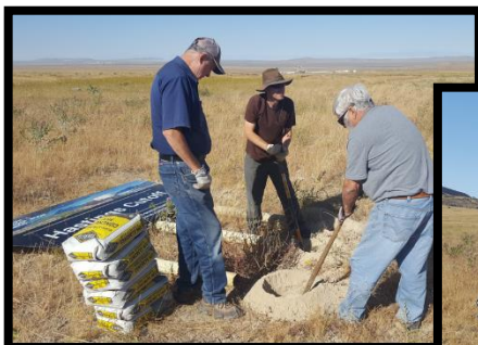
Dig post holes
