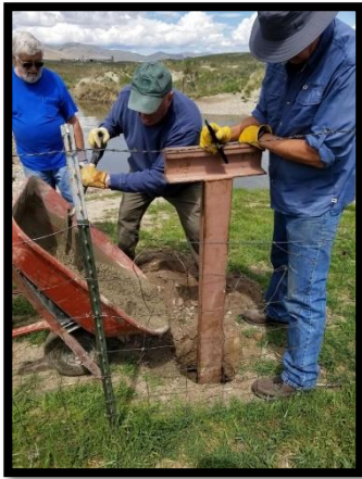
T-Post is leveled as cement is poured
