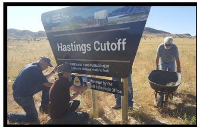
Cement poured into post holes
