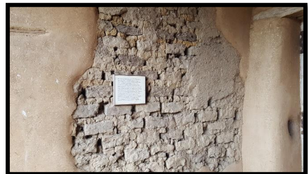
Adobe wall construction layers at Taos rancho
