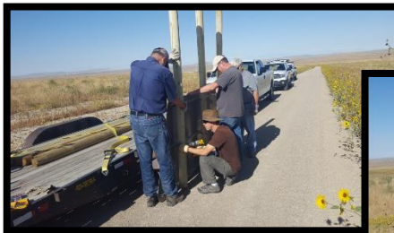
Attach new sign to poles
