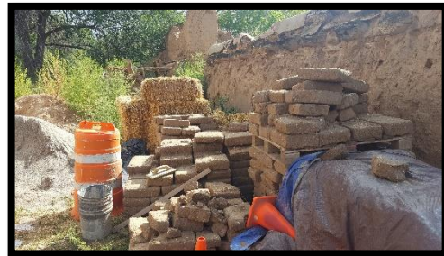
Adobe production area next to the church. Both bricks and plaster are made on site to keep the church strong. The church exterior plaster or mud is recoated each Spring.
